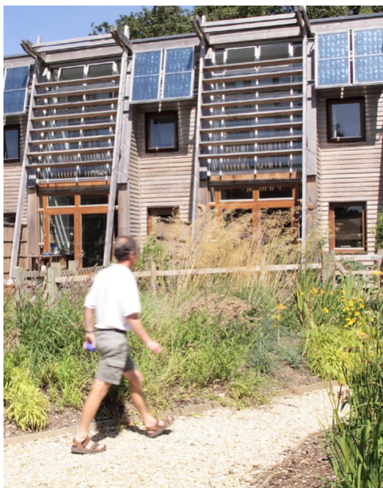
Figure 17: Low energy housing with passive solar design, including shading to prevent overheating in summer, and highly insulated thermal mass construction. Great Bow Yard, Langport, Somerset
